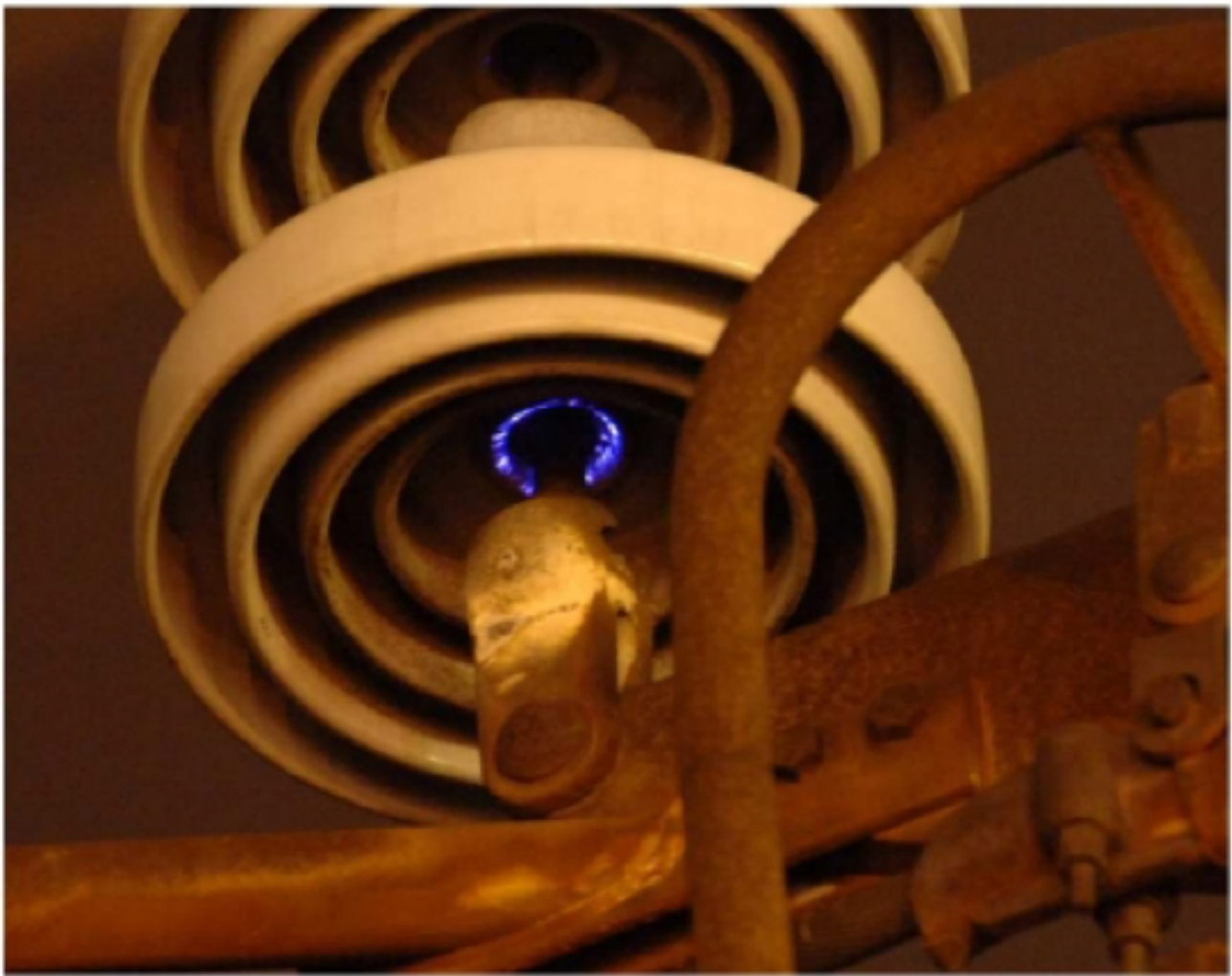
Streamer Corona in bottom of Insulator
